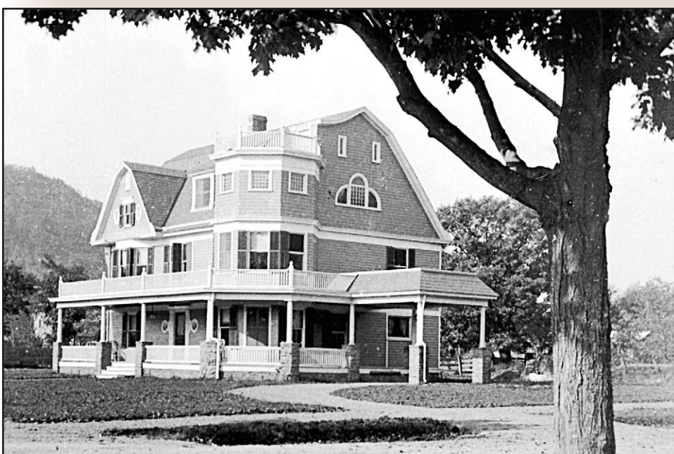
1898: Complex roof forms, wall textures and color variations are typical of the Queen Anne Victorian style. A porte-cochere originally extended from the right side of the house.
